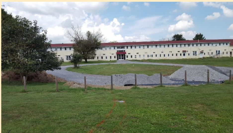
Driveway in progress
